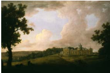
A View of Castle Howard, the West Front by William Marlow, c. 1770 Castle Howard
